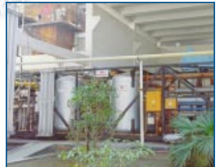
Along with other plant components, BOC Pakistan’s air treatment module (ATM) was transported from Hub to Lahore, Pakistan via truck. The ATM contains the equipment for chilling, dehumidifying, and purifying the process air before it enters the cold box.
