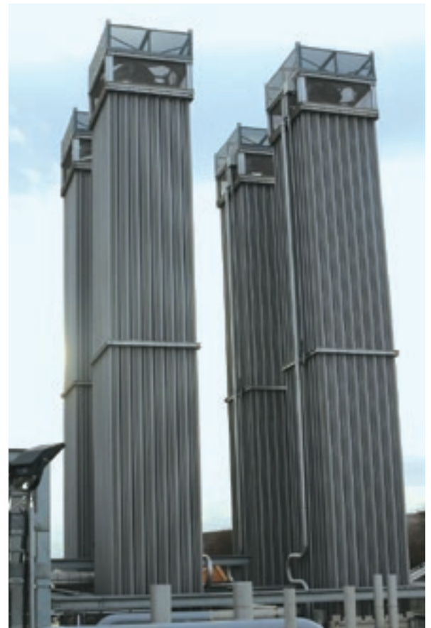
Ambient vaporizers with fog reduction modules
