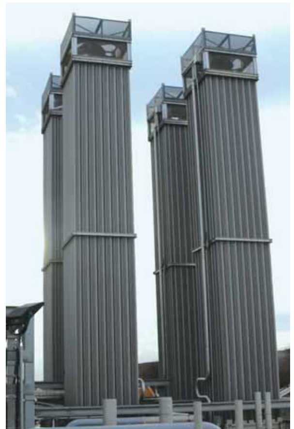
Ambient vaporizers with fog reduction modules
