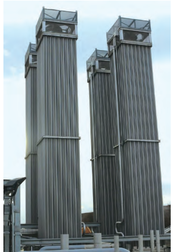
Ambient vaporizers with fog reduction modules
