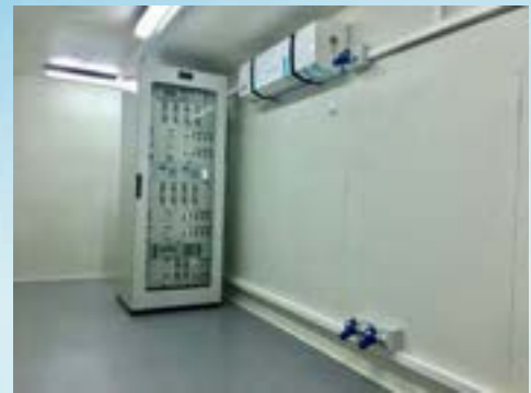
SHIPABLE ISO CONTAINER CONTROL ROOM AIR CONDITIONING AND INSTALLED ANALYSERS WITH LIGHTING, POWER, SOUND PROOF DOORS AND CLADDING
