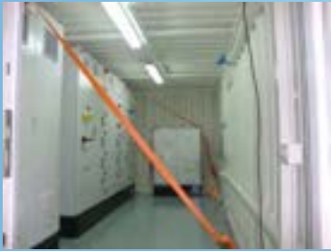
POWER DISTRIBUTION MCC SITE POWER DISTRIBUTION INSIDE A MODIFIED AND AIR CONDITIONED ISO CONTAINER
