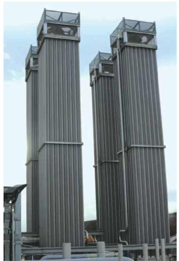
Ambient vaporizers with fog reduction modules
