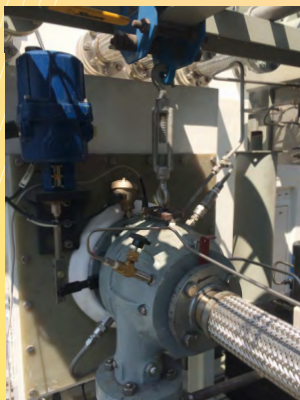
ACD TURBINE WITH LUBE OIL AND SEAL GAS SYSTEMS
